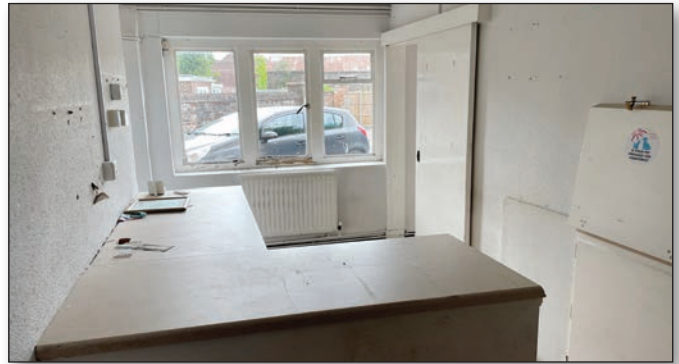
Former Vets' Reception Area
