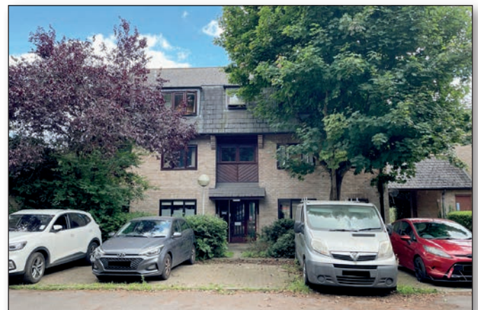
Rear of the Building
