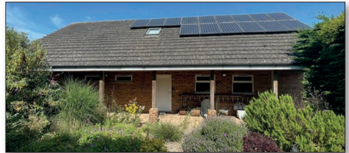
Side View of the Garage Building
