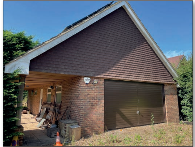
Front View of the Garage Building
