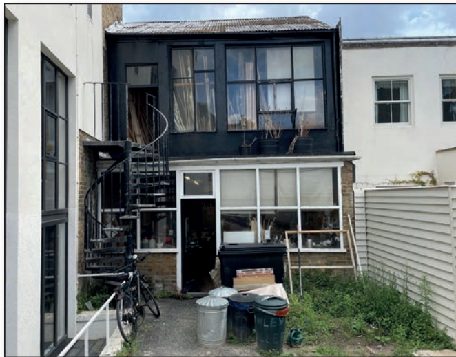
First Floor Workshop to Rear (Accessed via Spiral Staircase)
