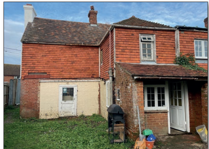
Rear of The Cottage
