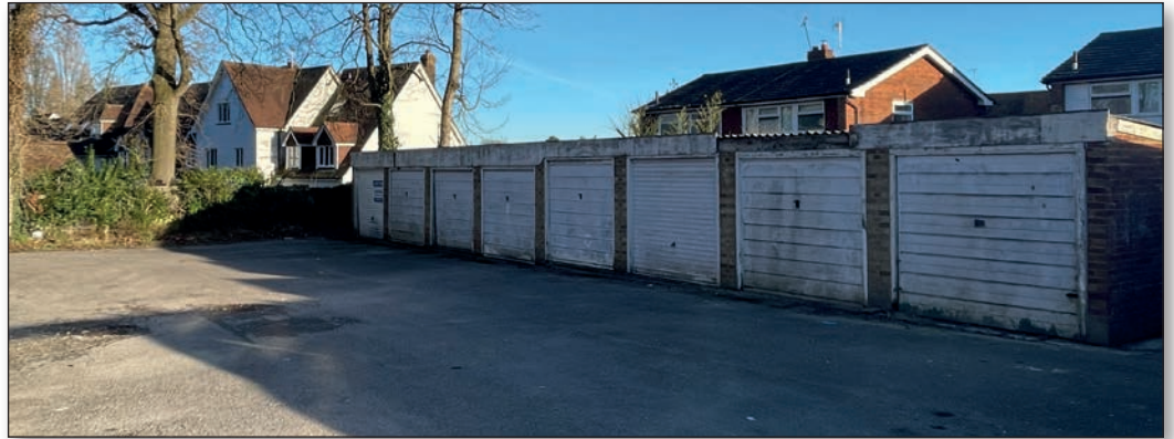
Above: View of eastern block of eight garages and forecourt
