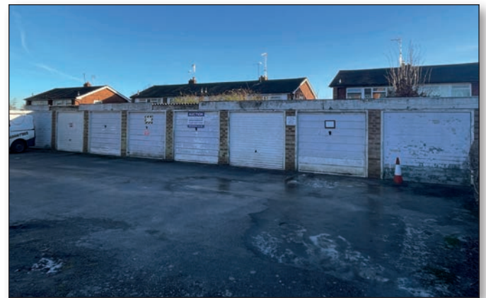
Above: View of western block of eight garages
