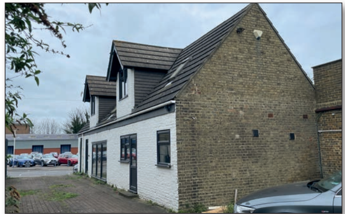
Offices in need of improvement
