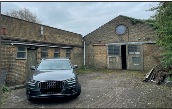
Courtyard and rear workshop
